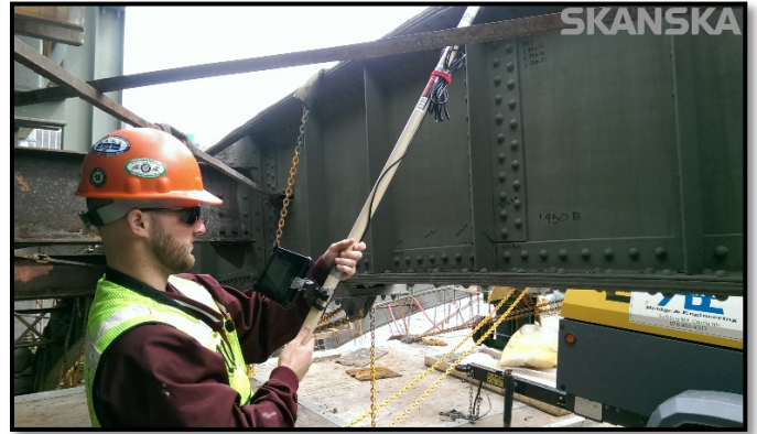
DPI-7SR & range pole on site at the Longfellow Bridge.
