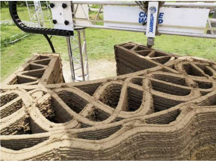
Figure 26: Italian company WASP has built one of the largest 3D printers in the world 125 . In the picture, the use of a clay-based 3D printer to build a sustainable house (“Tecla” project)
